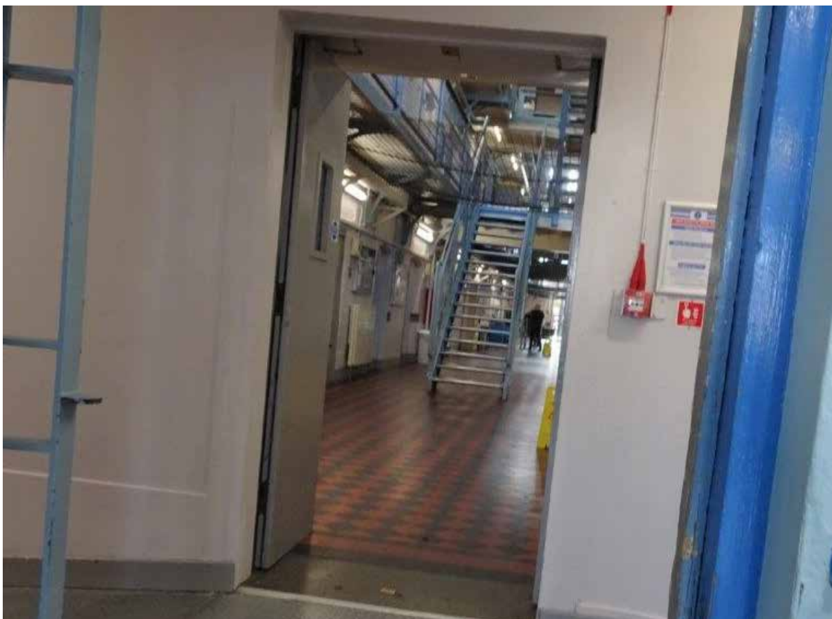
view of a residential hall
